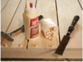
15 - If you are using plugs to hide the screws, I recommend a tapered plug cutter, like the Veritas Cutter from Lee Valley Tools. Glue the plugs in place with exterior waterproof glue, let dry, then cut off the excess with a chisel or Japanese saw, and sand smooth with a random orbital sander.
