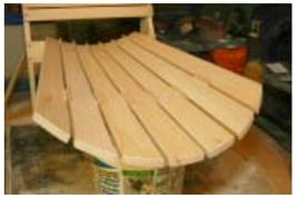
12 - Remove the back seat slat N. The back pieces can now be assembled, starting with the middle slat I, centered at the top on part H, and at the bottom, in the curve on part B. Use the drill hole locations centered on H & B and screw in place. I find it easier to level the chair as shown. I use 1/4" (6mm) spacers at the bottom, and 1/8" + 1/4" (3mm + 6mm) at the top.
